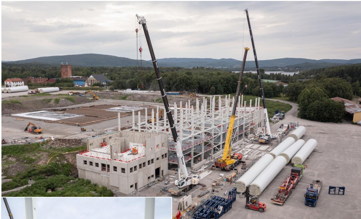
The building in the foreground is offices, the larger body of the building is for the production of mineral fertiliser, a total of approx. 2,000 sqm. On the large flat surface on the left, a 6,000 sqm salt storage is being built. Photos: Leif Wikberg
