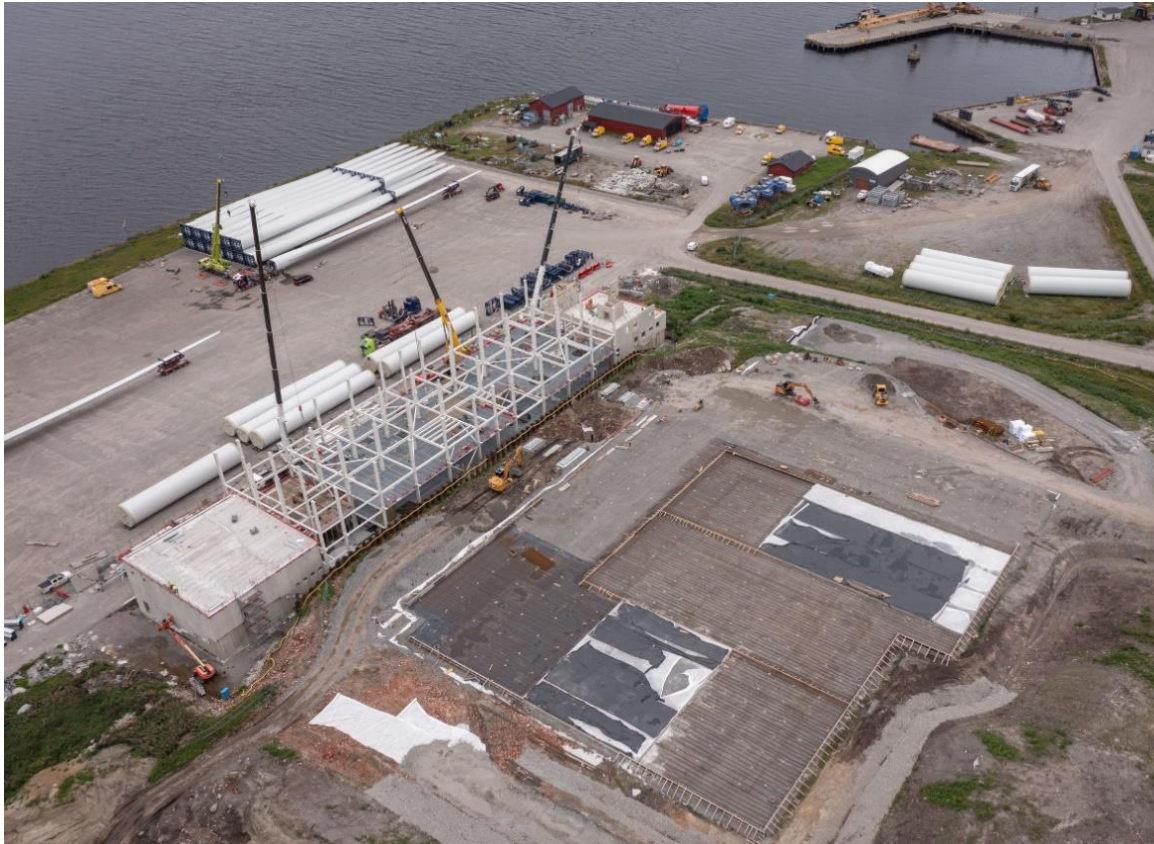
Cinis Fertilizer’s facility in the Örnsköldsvik municipality mid-August 2023. In the background is the port facility that the company will use. In the foreground, the floor for the salt storage is being poured. Frame assembly of the process plant is underway, and roofing has begun on the technology building on the far left. The large white elements are parts for wind turbines that are stored in the harbour area. Photos: Leif Wikberg
