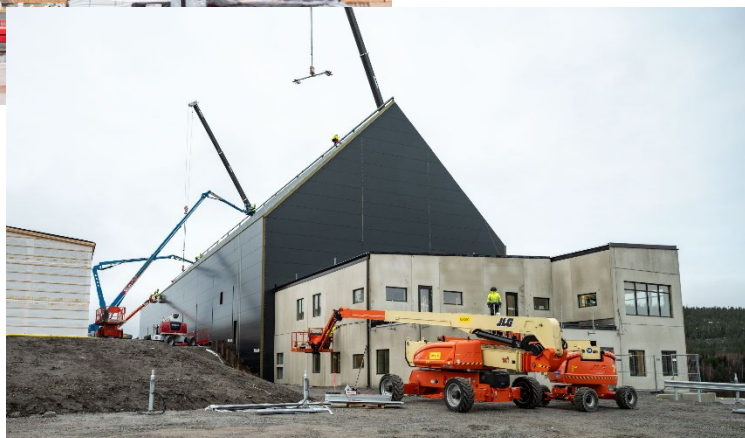
The walls of the salt storage are built in durable glue-laminated timber, a construction material produced from a renewable raw material that produces the least possible climate impact throughout the entire life cycle.
