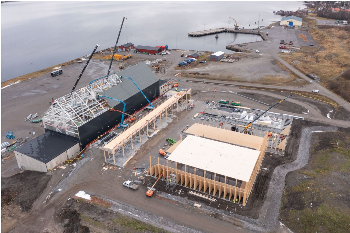
At the beginning of November, the process building on the left in the picture, is being roofed. The work should result in a waterproof house before the end of November. The salt storage in the center of the image will be approximately 6,000 square meters and will hold the four types of salt that will be handled in the process, the inputs sodium sulphate and potassium chloride and the end products potassium sulphate and sodium chloride, respectively.
